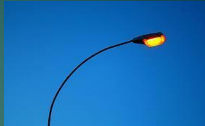
Figure 1: Standard high pressure sodium [1]
